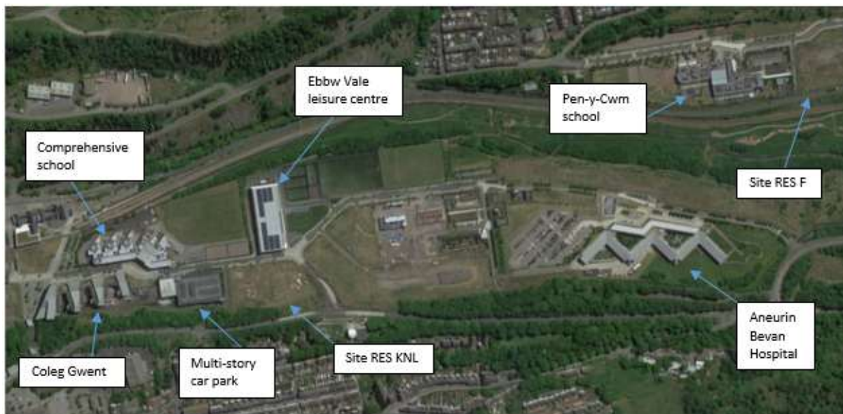
Map 4: Ariel image of the Works Site in Ebbw Vale on which both top sites are located
